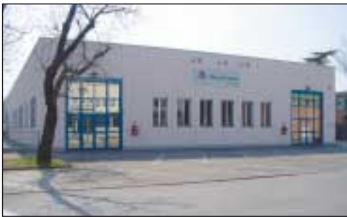
Production premises for Power products
