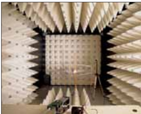
Anechoic room - R&D building
