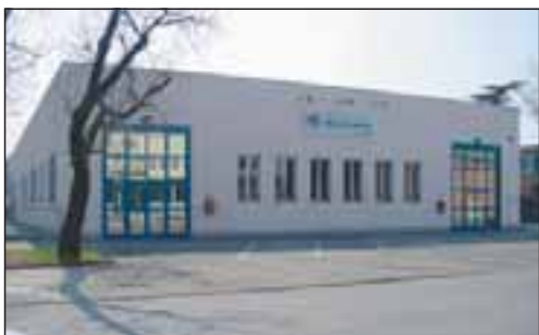
Production premises for Power products
